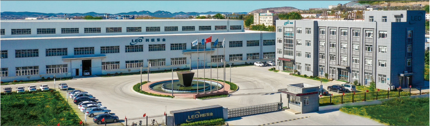
Pump Manufacturing Base for Petrochemical Industry
